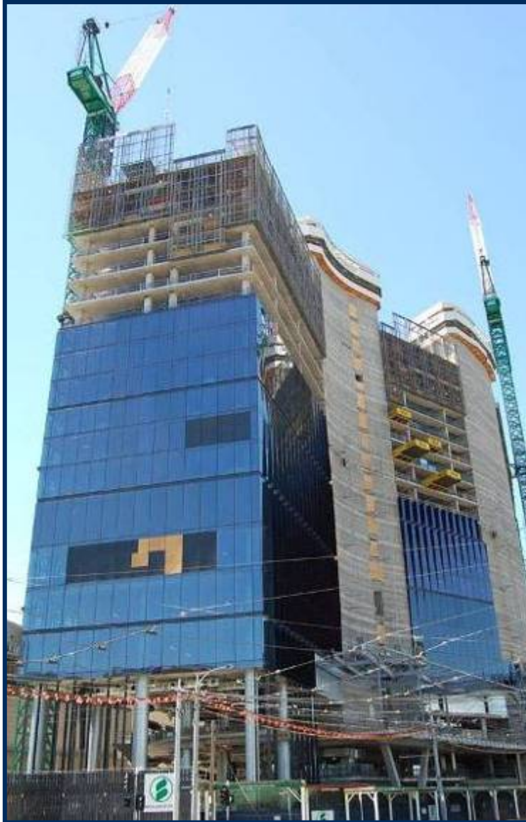
Construction of Third Hotel
