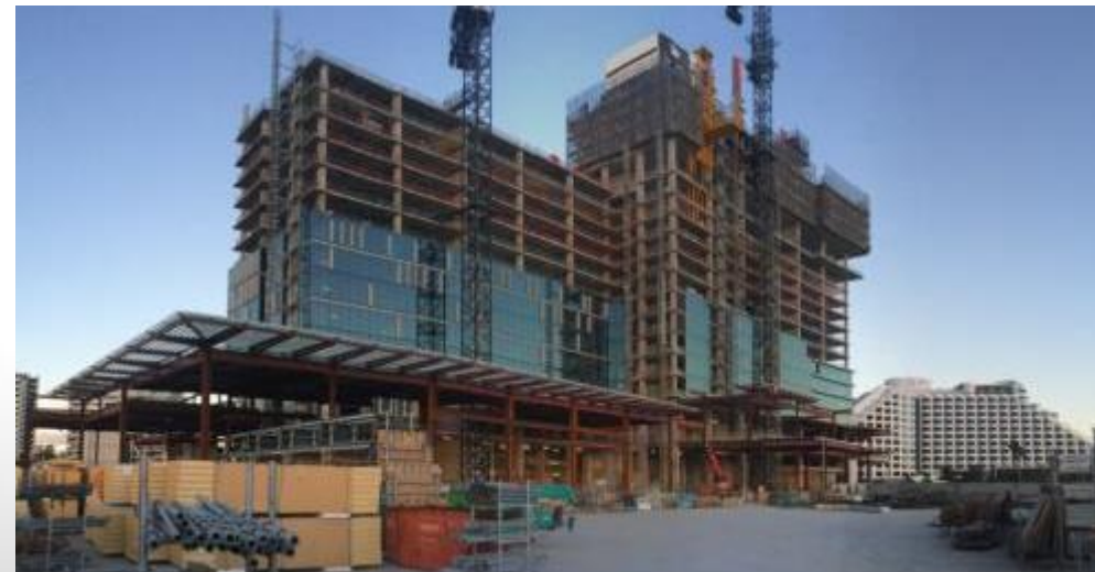
Construction Progress | End of June 2015
